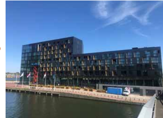
Hotel Jakarta, Amsterdam, 32 m 2+8 Floors, CLT – 3D modules Completed in 2018
